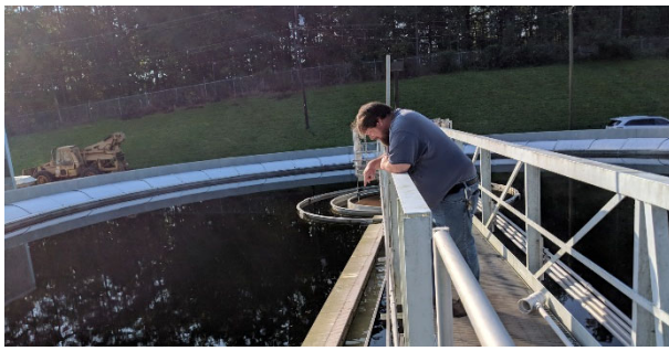
A utility mechanic inspects a mechanical arm on the Wastewater Treatment Plant's clarification tank, which sweeps the water surface of large organics and trash.
